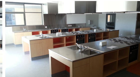
Custom Stainless Steel fabricated benchtops with integrated radiused bowls, Custom Stainless Steel splashback panels
