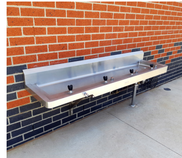
(L-R) Multiple Britex S.S. Pattern 6 Disabled Drinking Trough at 2000mm long pre-plumbed with four Remote Push Button Bubblers.
