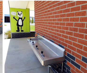
(L-R) Multiple Britex S.S. Pattern 6 Disabled Drinking Trough at 2000mm long pre-plumbed with four Remote Push Button Bubblers.
