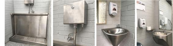
(L-R) Stainless Steel Mens Bathroom Fit Out including Stainles Steel Sanistep Urinal with Stainless Steel Push Button Cistern and Britex Flush Pipe Kit, Vandal Resistant Grandeur Hand Basin with Britex Eco Timed Flow Push Button Tapware and Framed Mirror, Accessible Bathroom Fit out with Accessible Hand Basin, Compliant Lever Activated Tapware, adjacent Stainless Steel Shelf and Framed Mirror 450x1000mm.
