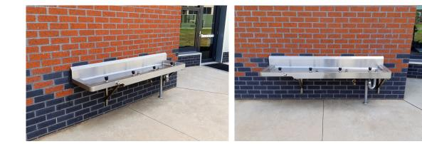
(L-R): Multiple Britex S.S. Pattern 6 Disabled Drinking Troughs at 2000mm long pre-plumbed with four Remote Push Button Bubblers.
