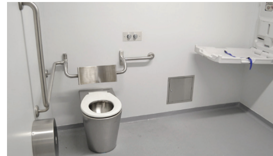
(L-R) Stainless Steel Toilet fit out including Disabled Pan with Toilet Seat, Backrest, Disabled Toilet Paper Holder, In Wall Cistern with Disabled (raised) Buttons, Sanistep Urinal complete with our Smart Sensor Flush, Disabled compliant Polished Stainless Steel Mirror, Disabled Hand Basin complete with Anti Vandal Tapware and Stainless Steel Security Shelf.
